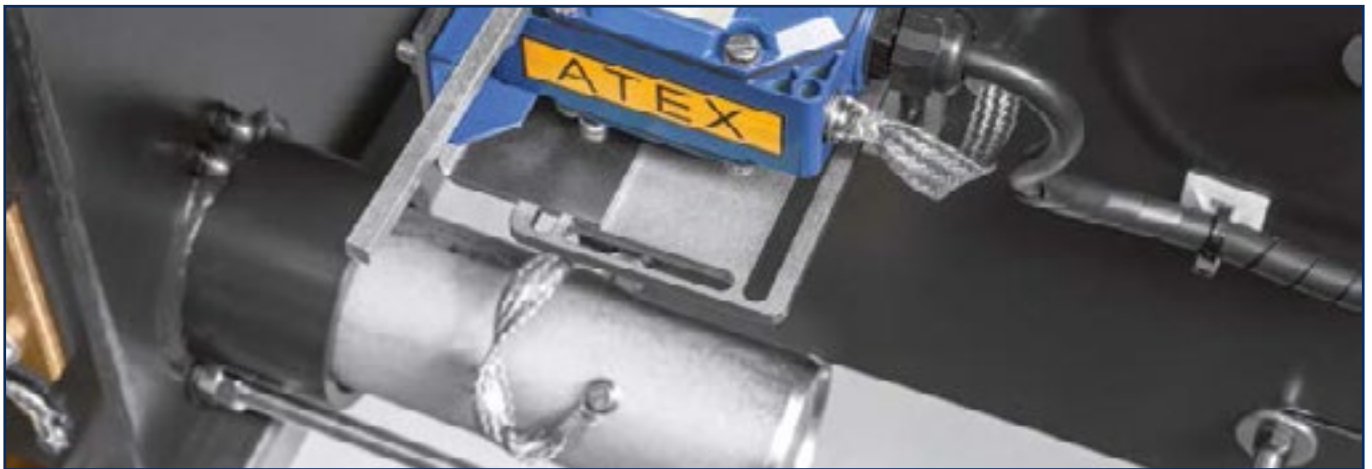
Potential equalisation using earthing strap
