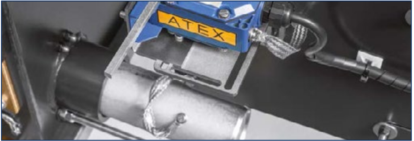
Potential equalisation using earthing strap
